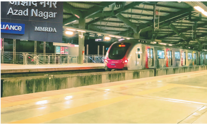
Azad Nagar Metro Station - 1.2 Km
