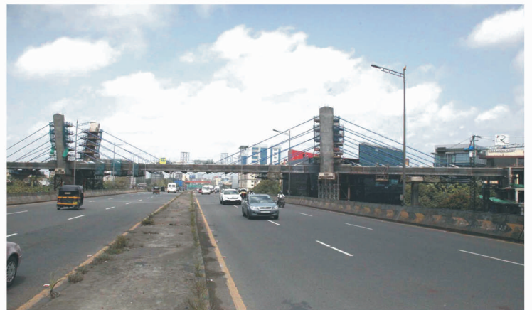
Western Express Highway - 1.5 Kms
